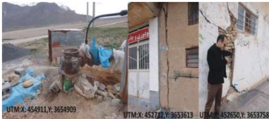
Fig. 2. Numerous fractures and cracks in the residential area
